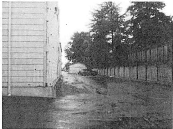
Southern view of the subject along the west property line, from the northwest property corner.
