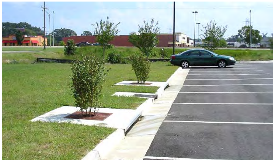
Tree Well Filters (by Filterra )
