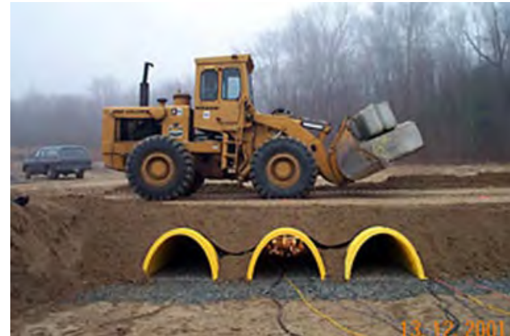
Subsurface Storage Chambers (by StormTech )
