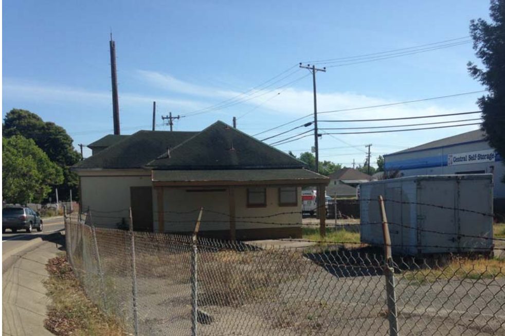
Figure 4-3 View from Sherman Street of Existing Yard House Building
