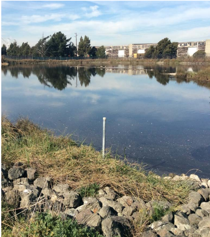
Figure 6 - Stand pipe from aeration system
