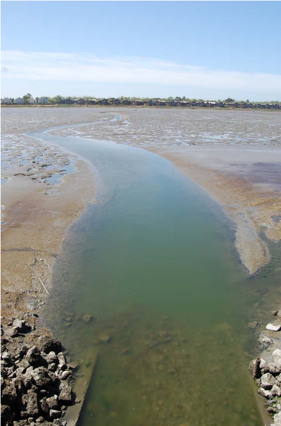
Outfall at San Francisco Bay San Leandro Channel
